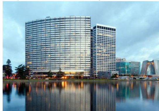
View of KP Northern California Pharmacy Operations Office Building at Lake Merritt
